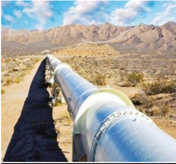
Pipe Laying Contractors
